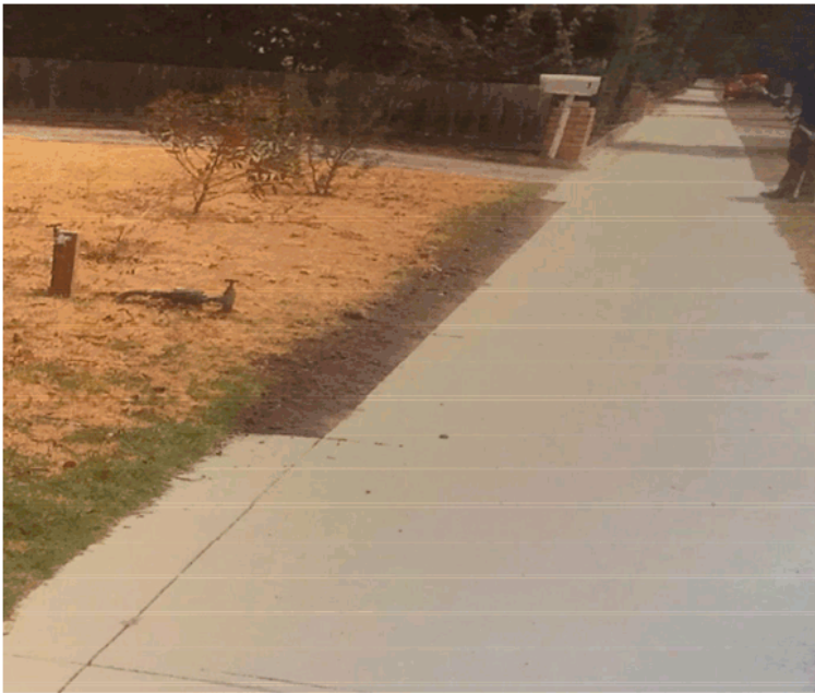
South-east end of Sharan Avenue showing selective removal of 'failed strips' in early 2013. Many potential future risk hazards ( now failed strips ) left in place.
